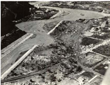
This aerial view of the 1938 flood from above Victory Blvd, shows breaches in paved levees in and below a sharp curve in channel alignment. Source: USACE, 1938.
